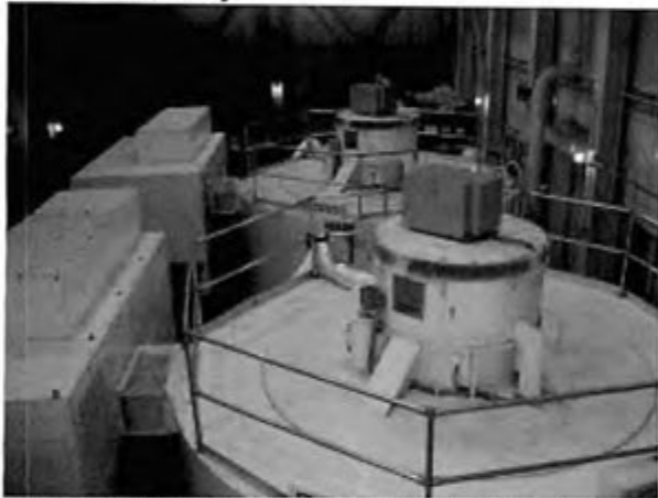
These are the two 10 MW vertical axis impulse Pelton-type turbine generators that generate electricity by using the flow of water. The plant is built against a very steep mountain below a river and lake where there is a dam actually on Terror Lake.
